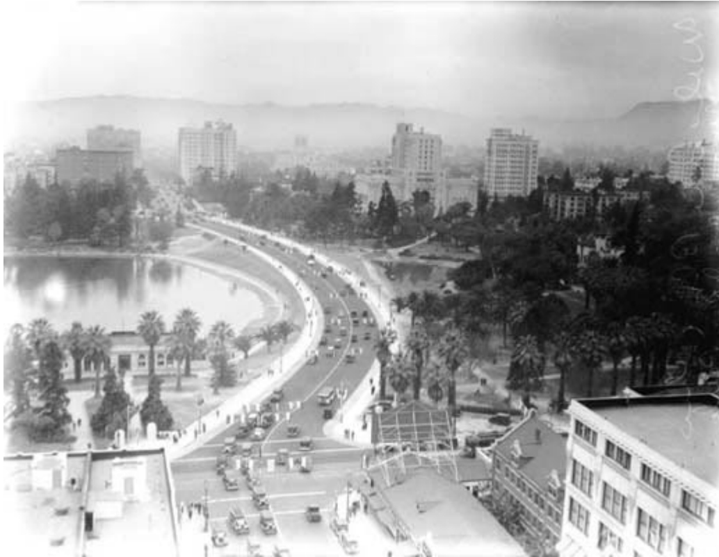
The Wilshire Extension Severed Westlake
